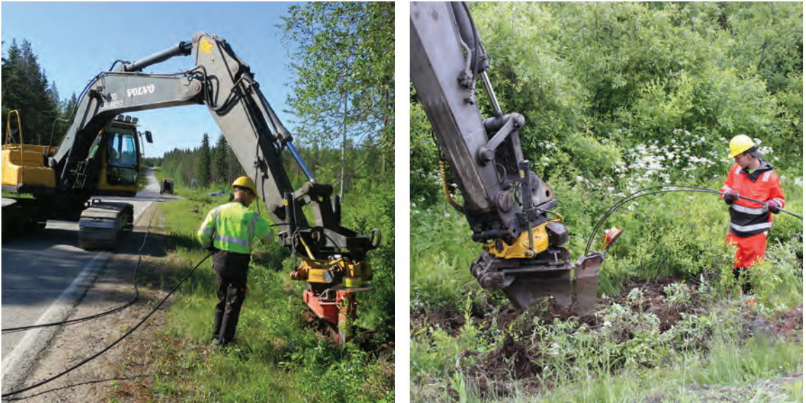
Figure 7.10. Examples of cable ploughing.
