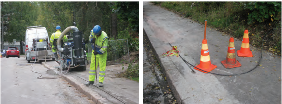
Figure 7.13. Microtrenching.
