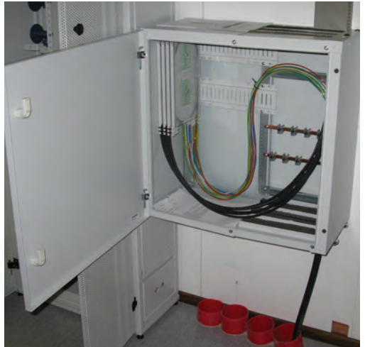
Figure 4.25. Installed indoor joint closure and splice cabinets.
