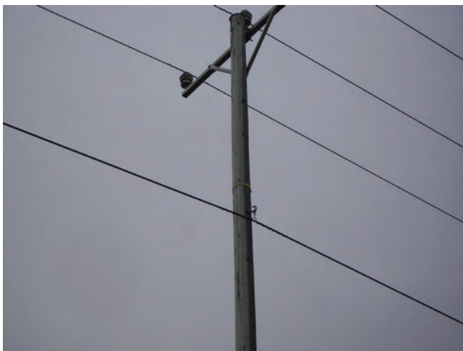
Figure 7.15. Installation of all dielectric self-supporting (ADSS) aerial cable.
