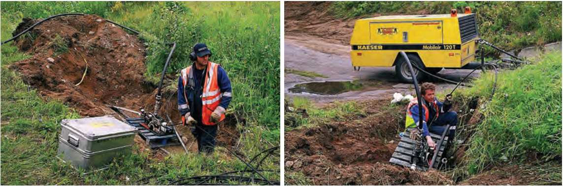
Figure 7.5. Cable blowing.
