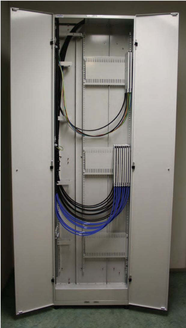
Figure 4.25. Installed indoor joint closure and splice cabinets.
