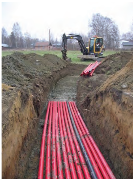
Figure 7.3. Installation of duct system.
