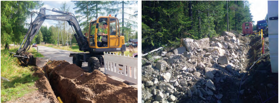
Figure 7.8. Installation of direct burial cables.
