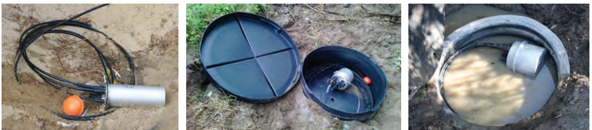
Figure 4.22. Installed outdoor joint closures.
