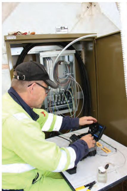
Figure 8.3. Splicing of optical fibres with a fusion splicer.
